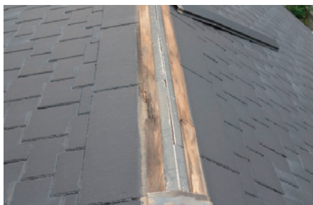
写真7: 棟の破損
